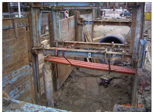
Blick in Baugrube
